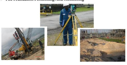
In places where it is required to drive piles for foundation and other engineering purpose, we can position the piles to within a few millimetres accuracy. This feat can be achieved using total station with given coordinates to set out this position and we also monitor the piles for verticality during piling. We also provide survey service for shore protection piling and pile sheet monitoring.
